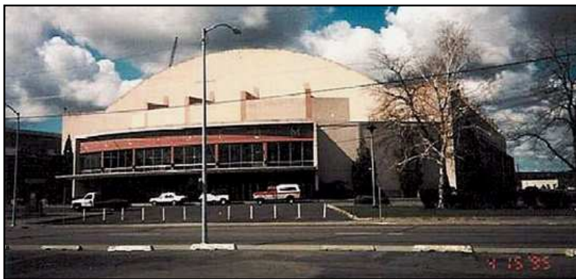
Spokane Coliseum: Broke ground, September 28, 1953; Opened December 3, 1954; Closed, Spring 1995 (40 years); Demolished, Spring–Summer 1995. Note that the date of this photo is April 15, 1995, so it is one of the last photos.
