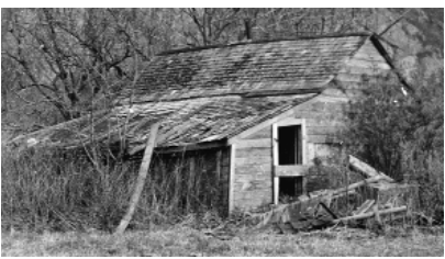
For many years the Chapman house remained vacant and eventually crumbled. These photographs show the house probably fifteen years or so after it was left to the elements.
